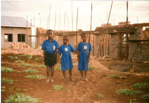
Construction of St. Gertrude School -30 yrs. ago
